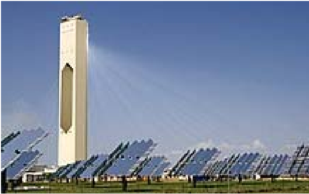
Solar thermal power plant with a field of heliostats and a central solar power tower
